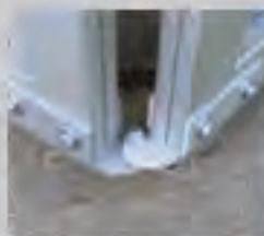
1/4 in. plate steel hinge system.
